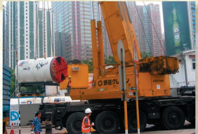
Baustelle in Hongkong, China / Jobsite in Hong Kong, China
