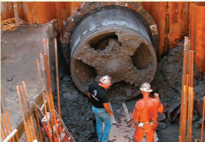
Baustelle in Seattle, USA / Jobsite in Seattle, USA
