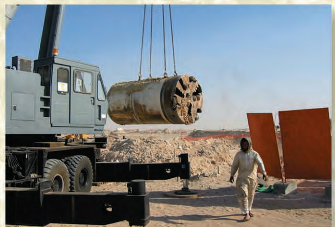
Bergung Bohrkopf aus Zielschacht, Abu Dhabi, VAE / Recovery of cutter head, Abu Dhabi, UAE
